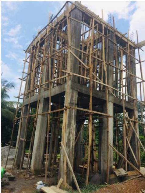
Water tower under construction
