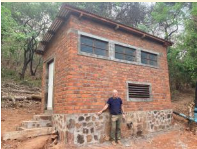
Newly built turbine house, Lwamba
