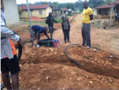
Laying pipework, Manowa
