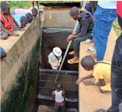
Measuring the Kuluva intake
