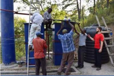
Installing the Clariwash filter, Kagando Hospital
