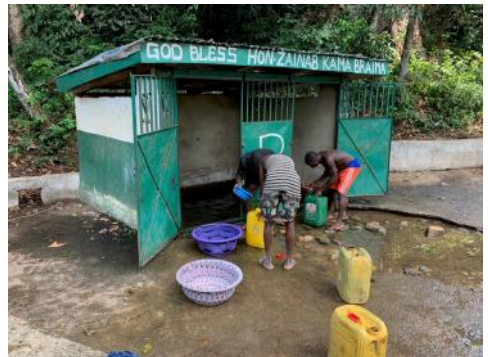
Existing spring, inadequate and often contaminated
