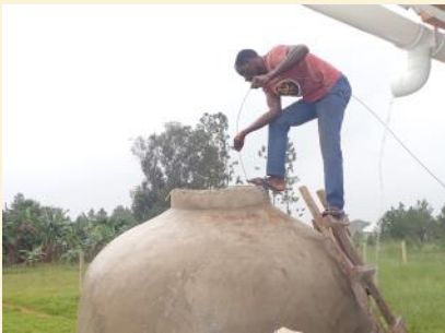
Removing the steelwork skeleton
