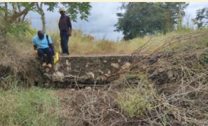
Spillway, Buhuri Dam
