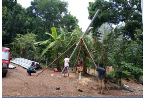
Borewell under construction
