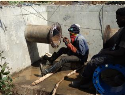
Welding a flange, Kuluva Hydro
