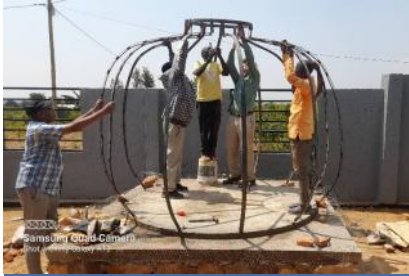
Building a 10,000 litre pumpkin tank
