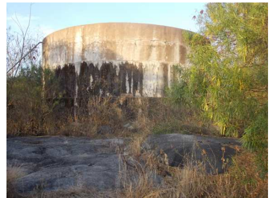
Existing water tank
