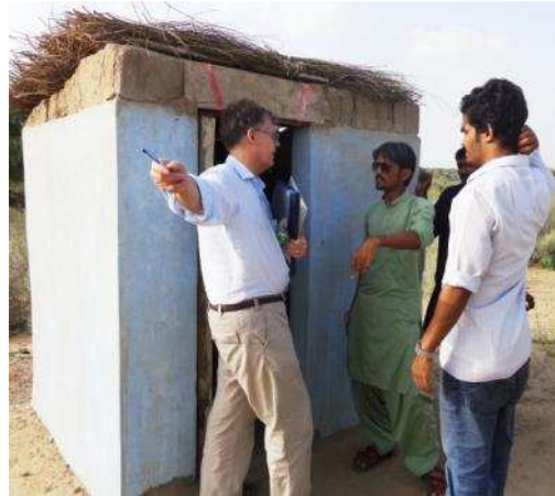
Latrine superstructure built by school
