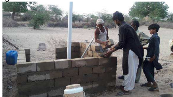
Latrine under constructionl
