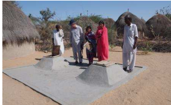
Cisterns with water catchment, Rana Tarai
