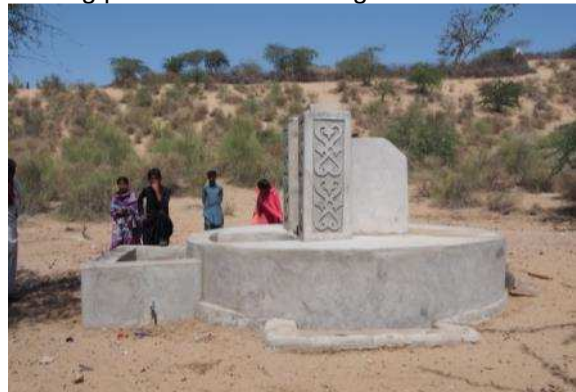
Repaired well, Bhemoo Bheel
